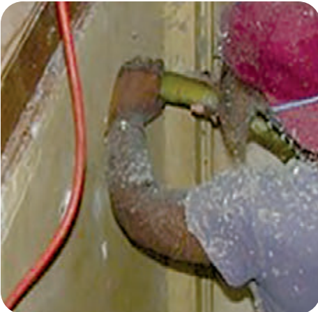
7. Dense pack stairway walls
