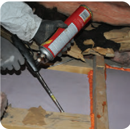
3. Ensure air sealing, if any, is completed
