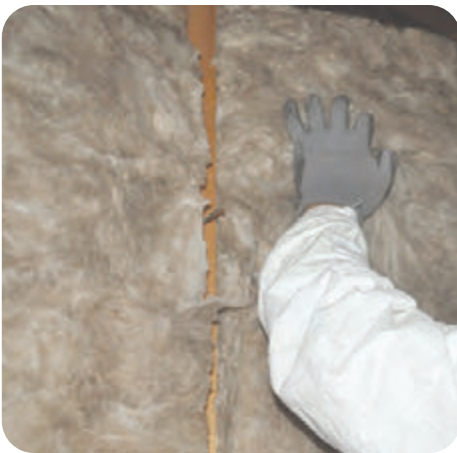
3. Install batts with minimal compression
