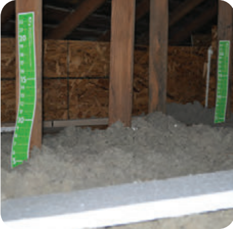
5. Depth rulers installed, 1 per 300 square feet
