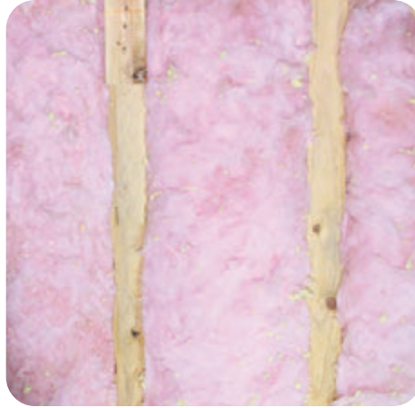
2. Cut batts for exact fit
