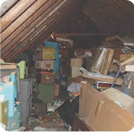
1. Remove stored materials
