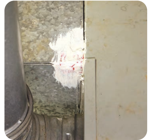
B-3. Apply mastic over the tape
