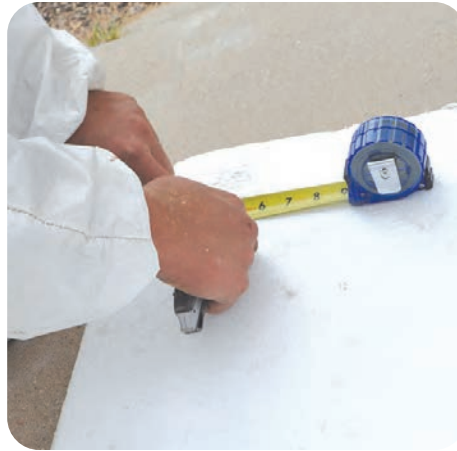
2. Cut blocking material to fit
