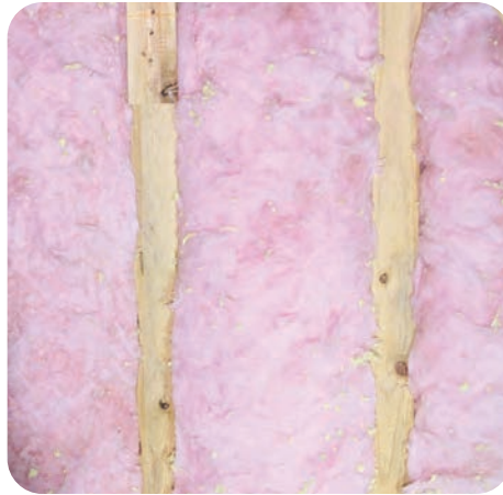
2. Cut batts for exact fit
