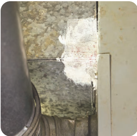
B-4. Push fiberglass mesh into the mastic
