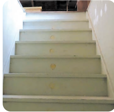
11. Plug access holes from blown insulation
