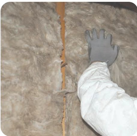
3. Install batts with minimal compression
